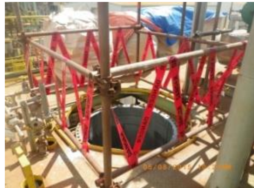
Proper- barricade on open column provided with post and railings.
