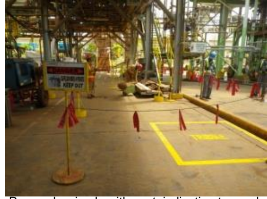
Proper- barricade with post, indication tag and access way.
