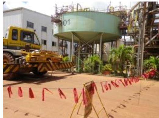
Proper- on going lifting activity with signage and watchman
