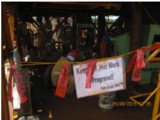
Proper- ongoing welding activity full barricade with indication tag
