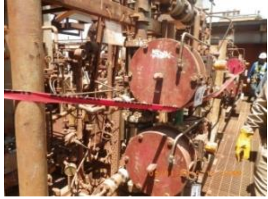
Improper – Should be caution tape only not danger tape. Not on going activity.
