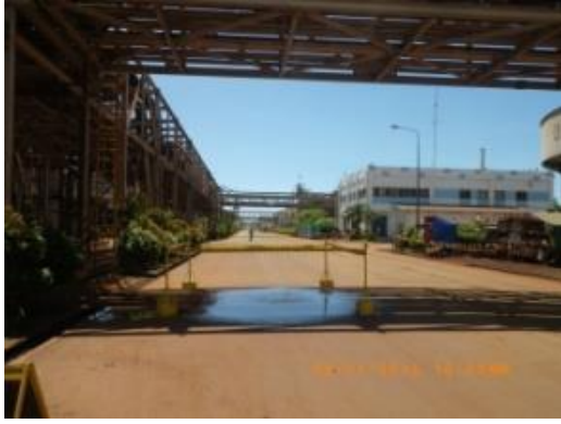
Improper – On going water leaking on pipe rack barricaded with caution tape should be danger tape.
